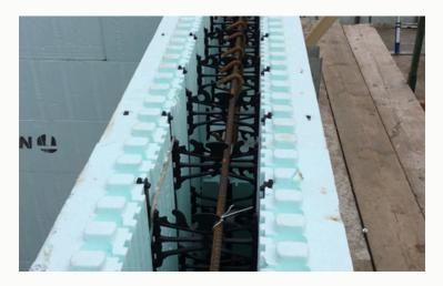
The product has excellent u-values; far exceeding building regulations and can be constructed very quickly. The walls of the building were constructed in less than two weeks, enabling the quick progress of other trades within the programme.
